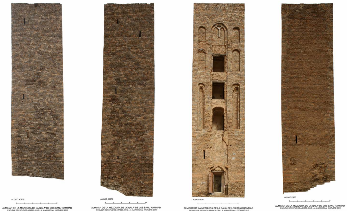
Figure 11. Photo rectifications of the façades of the minaret of the Qala of Beni Hammad, Algeria
