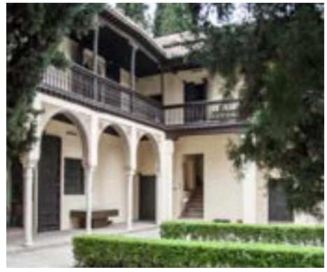
SOUTHERN PATIO, current state
